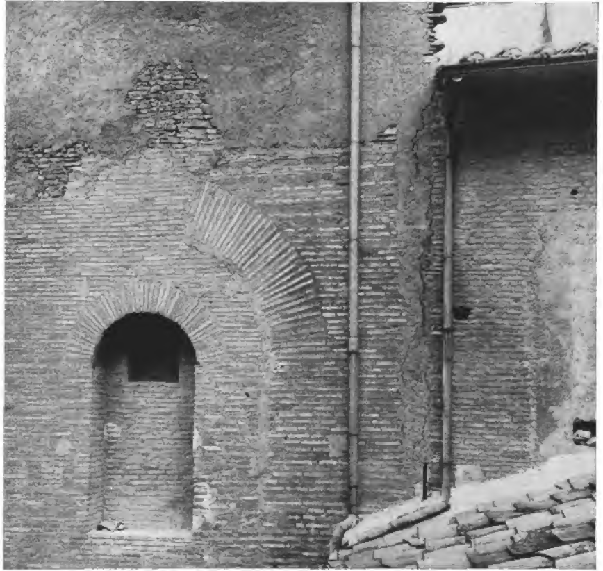
Fig. 143 — S. Lorenzo in Lucina. South end of west clerestorey, remains of Early Christian window arch (Photo: Sansaini).
